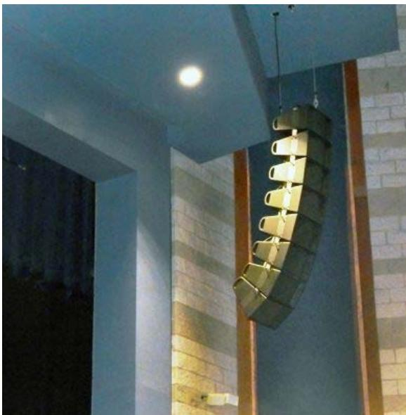
House PA is a flown L / R array composed of 16 Fulcrum Acoustics FL283 cabinets (8 per side) and 4 RCF 8006AS active subwoofers (two per side). The array is dead hung.
